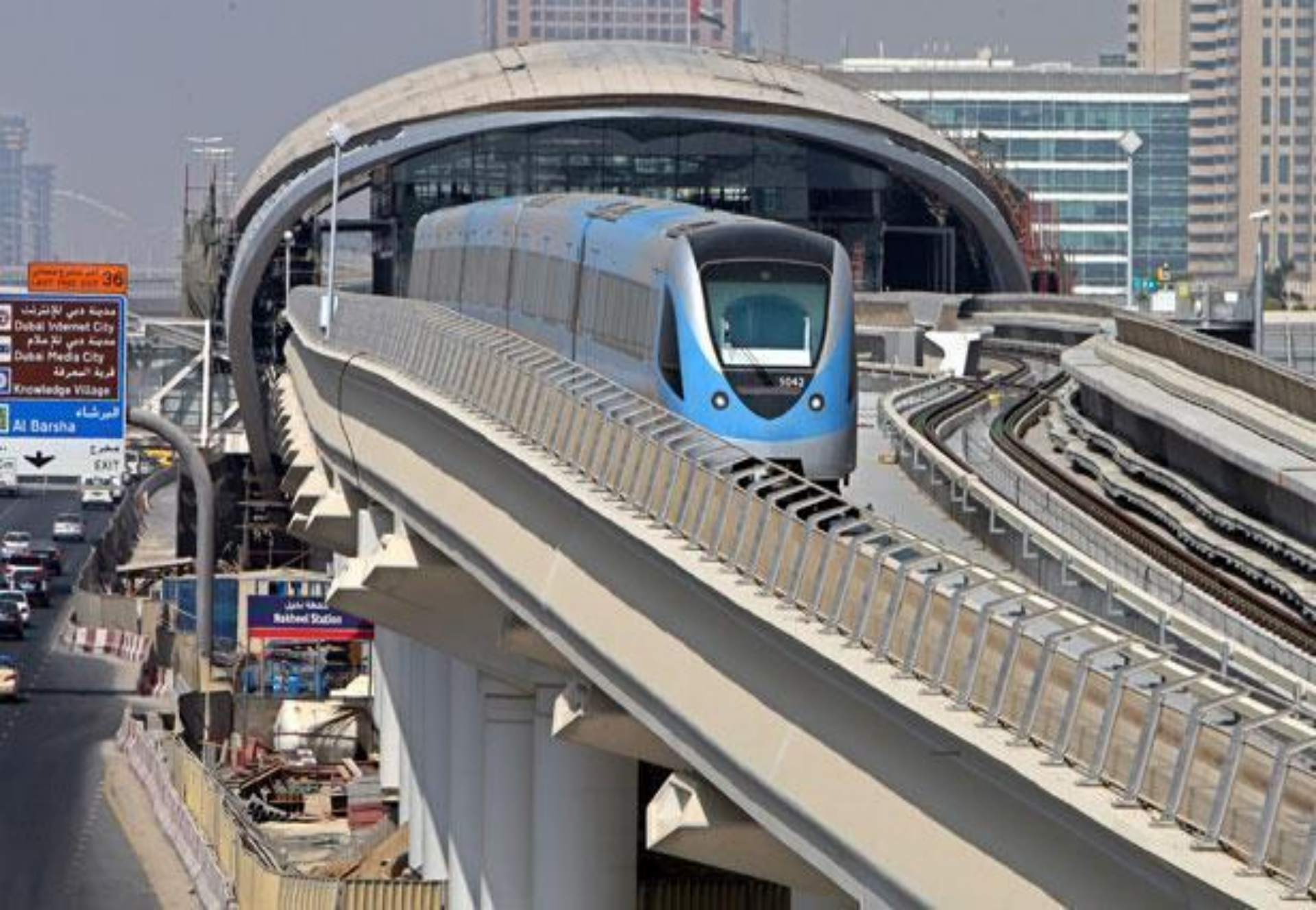
Dubai metro station
